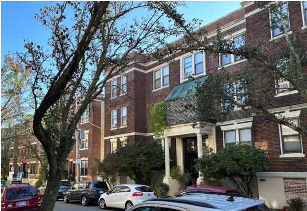
The Allston Brighton Community Development Corporation will retrofit and decarbonize 33 apartments on Carol Avenue in Brighton. (Courtesy of the Allston Brighton Community Development Corporation)
